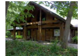
Exterior front view of the Nature Center. The entry hall has topographical maps, arrowhead display, tree house for the kids, live animal displays and a fireplace with seating. There is a full deck on the back of the building.
