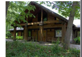
Exterior front view of the Nature Center. The entry hall has topographical maps, arrowhead display, treehouse for the kids, live animal displays, and a fireplace with seating. There is a full deck on the back of the building.
